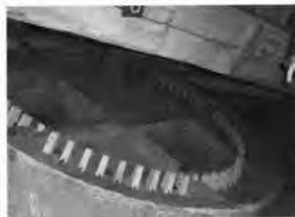
The brakewheel is a huge wooden gear mounted on the windshaft, fitted with wooden cogs made of hornbeam, each one individually mortised into the rim of the wheel.
