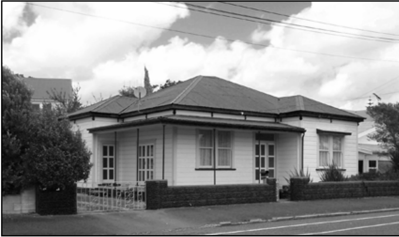
3 Ingestre Street, Wanganui, New Zealand
